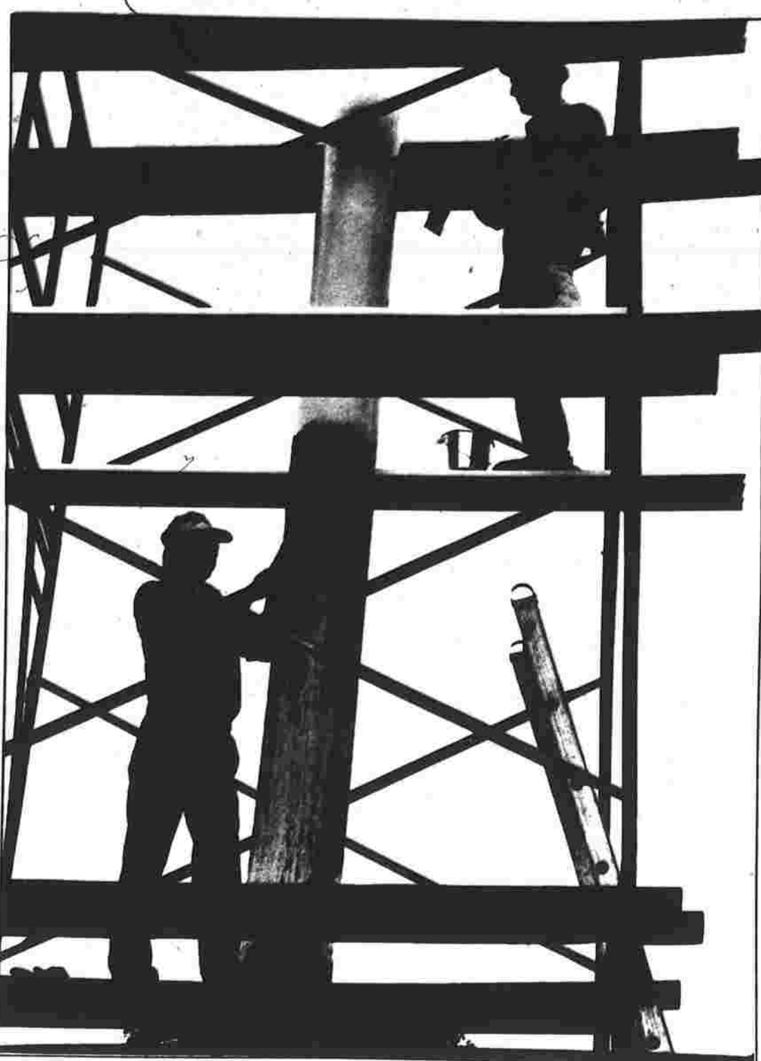
On the scaffolding
